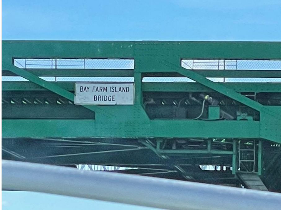
BAY FARM BRIDGE.
