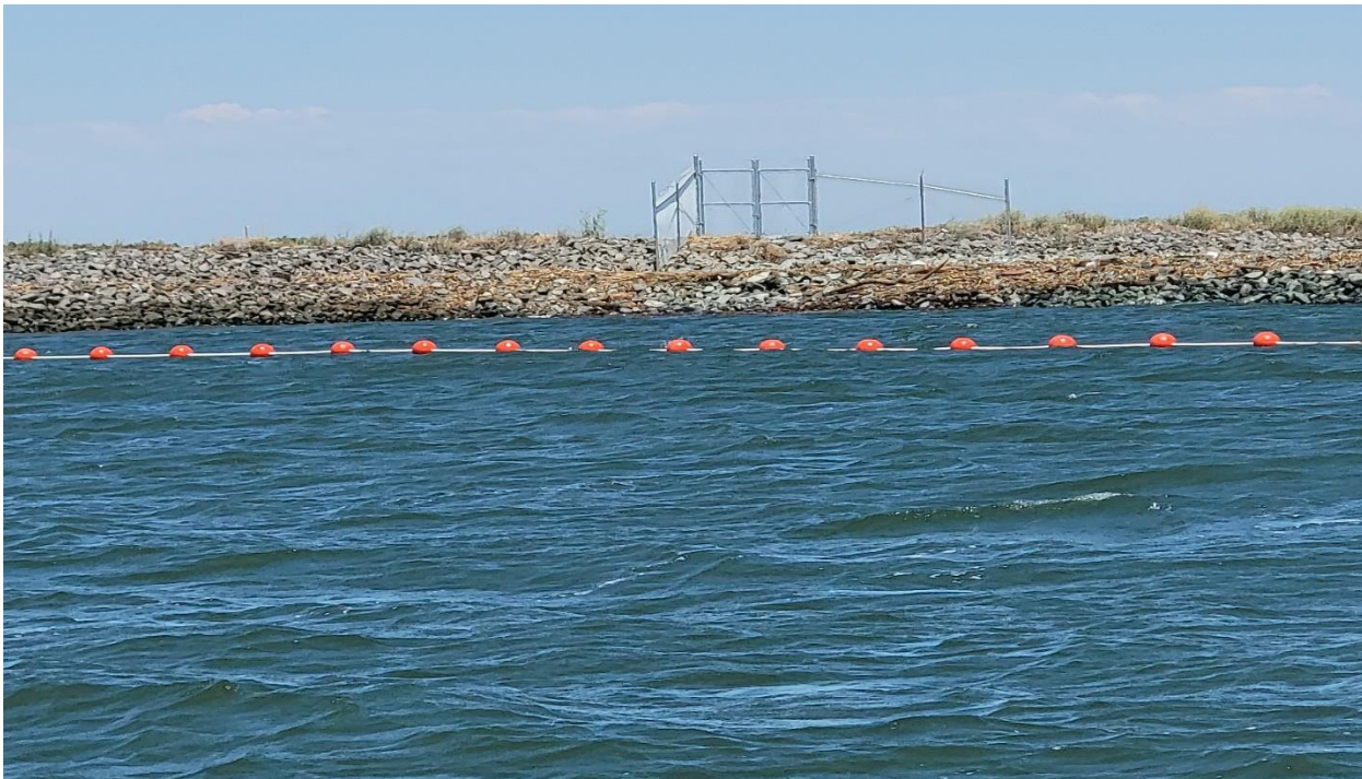
A picture showing barrier Buoys and warning sign on False River Temporary Rock Dam
