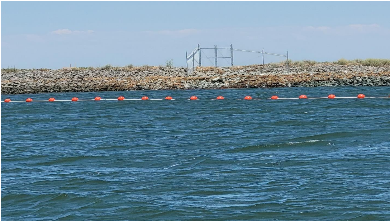
A picture showing barrier Buoys and warning sign on False River Temporary Rock Dam
