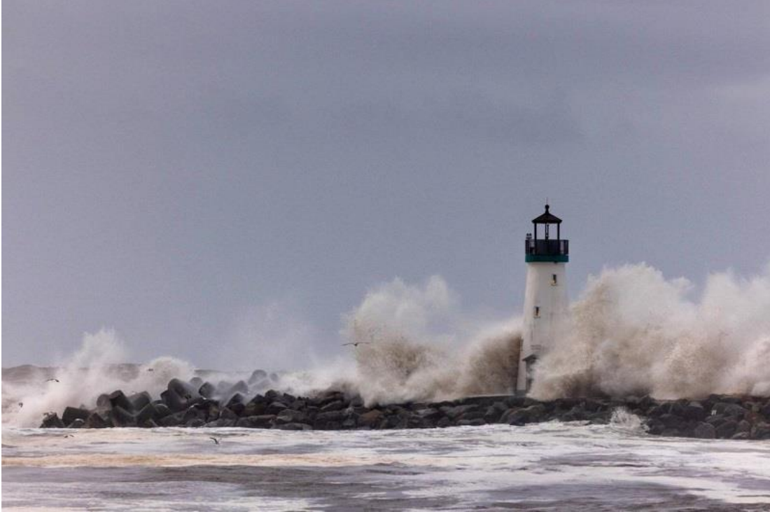
Santa Cruz Harbor West Jetty – New Year's Day 2023
