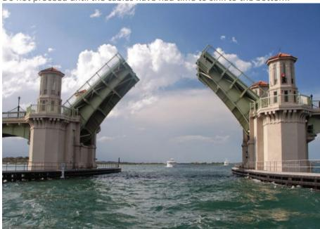
**Bascule Bridges** are the most common type of opening bridge you will encounter. The opening section has one or two leaves that tilt vertically on a hinge like doors being opened skyward.
