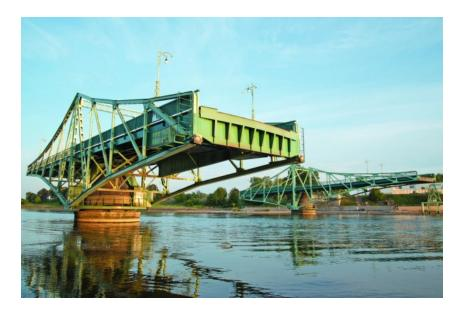
Swing Bridges have an opening section that pivots horizontally on a central hub, allowing boats to pass on one side or
