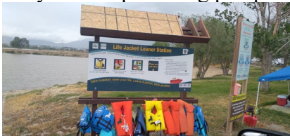
Life jacket station under construction 1 of 6
