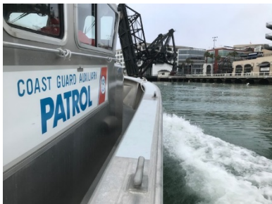
Checking on bridge maintenance in SF.
